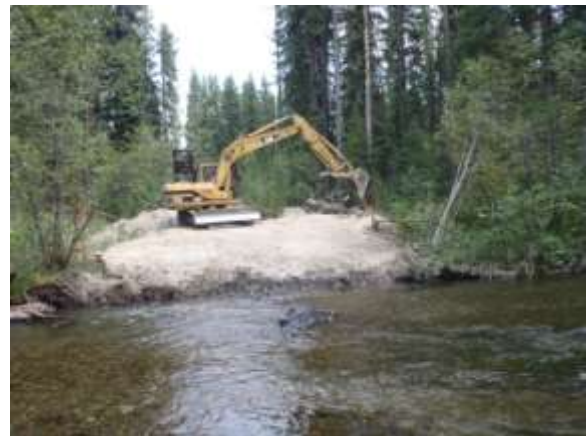
Bridge abutment removal at Cold Creek. Courtesy Photo.
